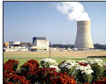
Grand Gulf Nuclear Generation Facility Port Gibson, MS
